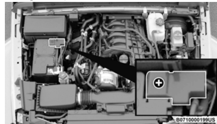
Positive (+) Battery Post – Gas Engine
